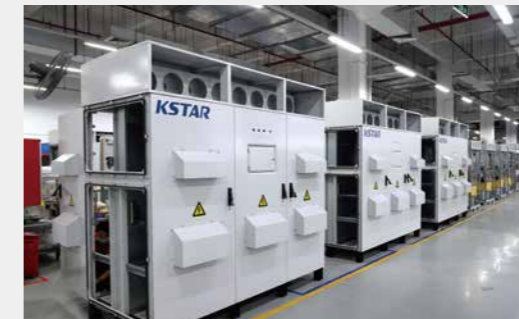
PV Assembly Workshop
